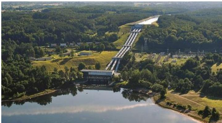
**Largest pumped storage power plant in Poland.** ZREW supplied three power transformers to ESP Żydowo, Poland's first and largest pumped storage power plant in Poland. The transformer ensures the plant can maintain a continuous supply of power to the Polish grid. The plant uses two natural reservoirs - Lake Kamienne and Lake Kwiecko - with an altitude difference of 82 meters.
